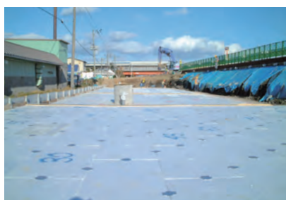
Construction example that was adopted as a load relief construction method due to embankment load on soft ground and suppressed the pull-in settlement of neighboring buildings
